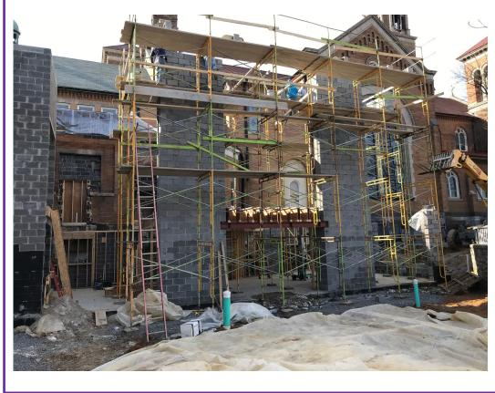
Our atrium is really beginning to take shape! In this photo, taken on February 28, you can see the concrete floor of the lower level, the completed elevator tower on the far left, the opening for the entrance between the front columns, and the steel support beam for the upper level floor joists. Now that demolition and site preparation is finished, we should run into fewer surprises, and construction should start progressing rapidly!
