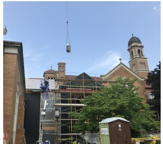
Rooftop A/C units being placed - May 29
