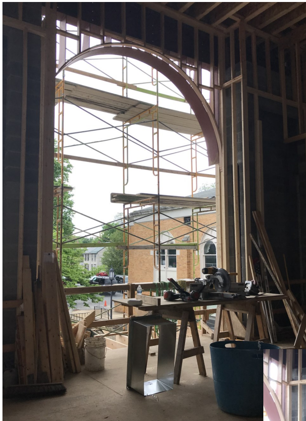
A view from the inside out - center window opening, upper level
