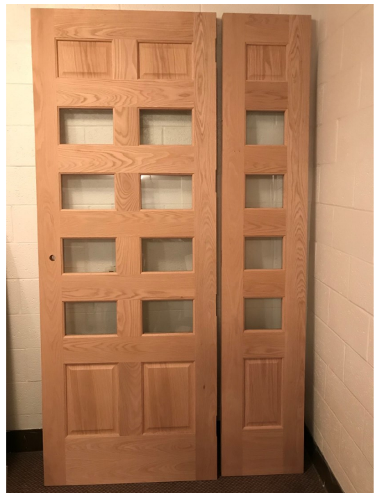
The new custom door. Both panels will open. The style mimics the current doors into the nave but with glass inserts. The wood will be stained to match the woodwork in the nave.
