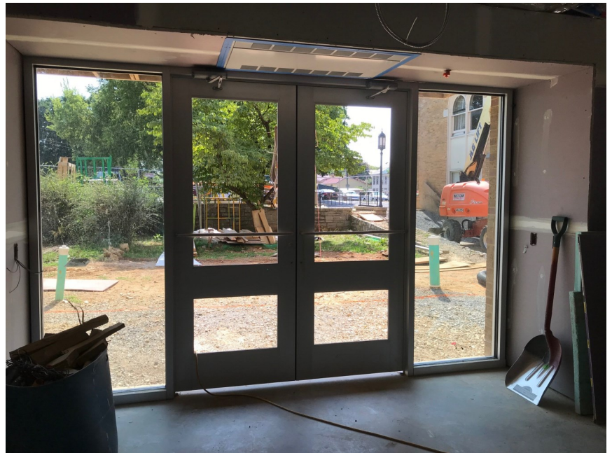
The view out of the new lower level lobby.
