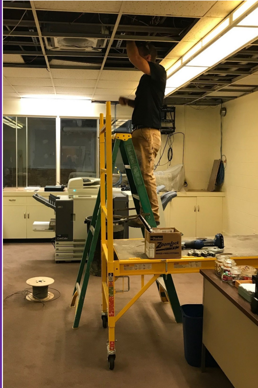
Installing the ceiling AC unit in the outer office.
