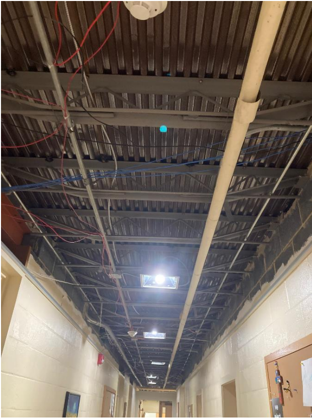
Christian Ed hallway ceiling - lower level - after demo!
